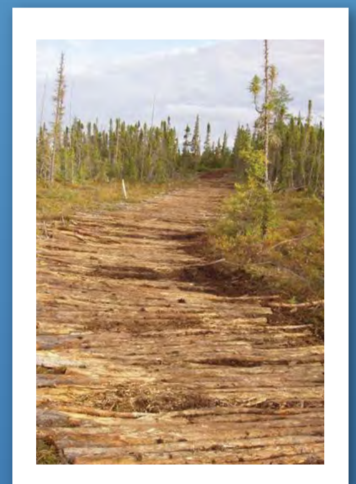
Corduroy Road - minimizes degradation of the land when moving drills
