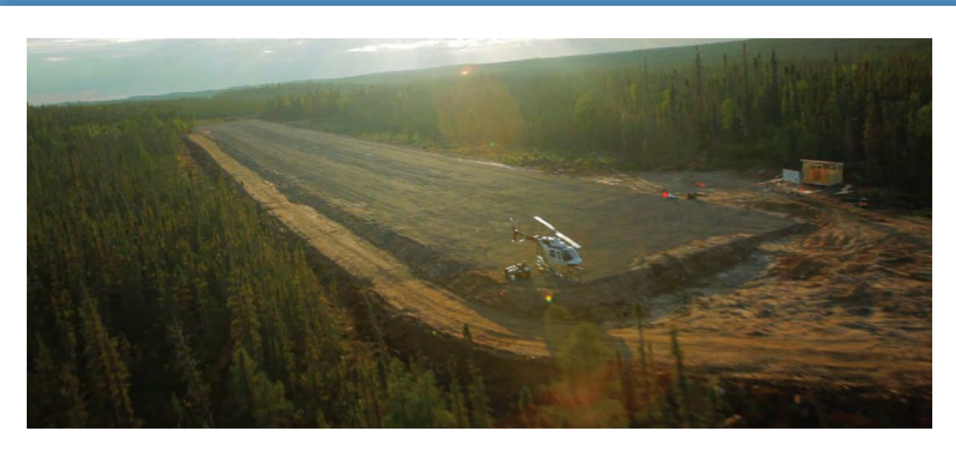
Thor Lake airstrip - land reclamation of legacy exploration; existing rock debris left on site was used in building the airstrip
