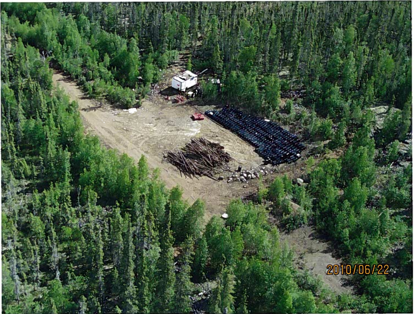
MV2010G0001 - Avalon Rare Metals Inc. - Thor Lake Trees that will be utilized for corduroying, fuel cache and Foraco tracked drill.
