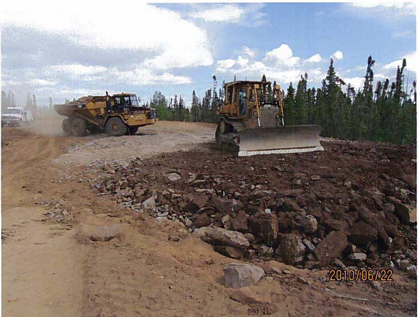
MV2010G0001 - Avalon Rare Metals Inc. - Thor Lake Rock truck and dozer working at the East end of the airstrip.
