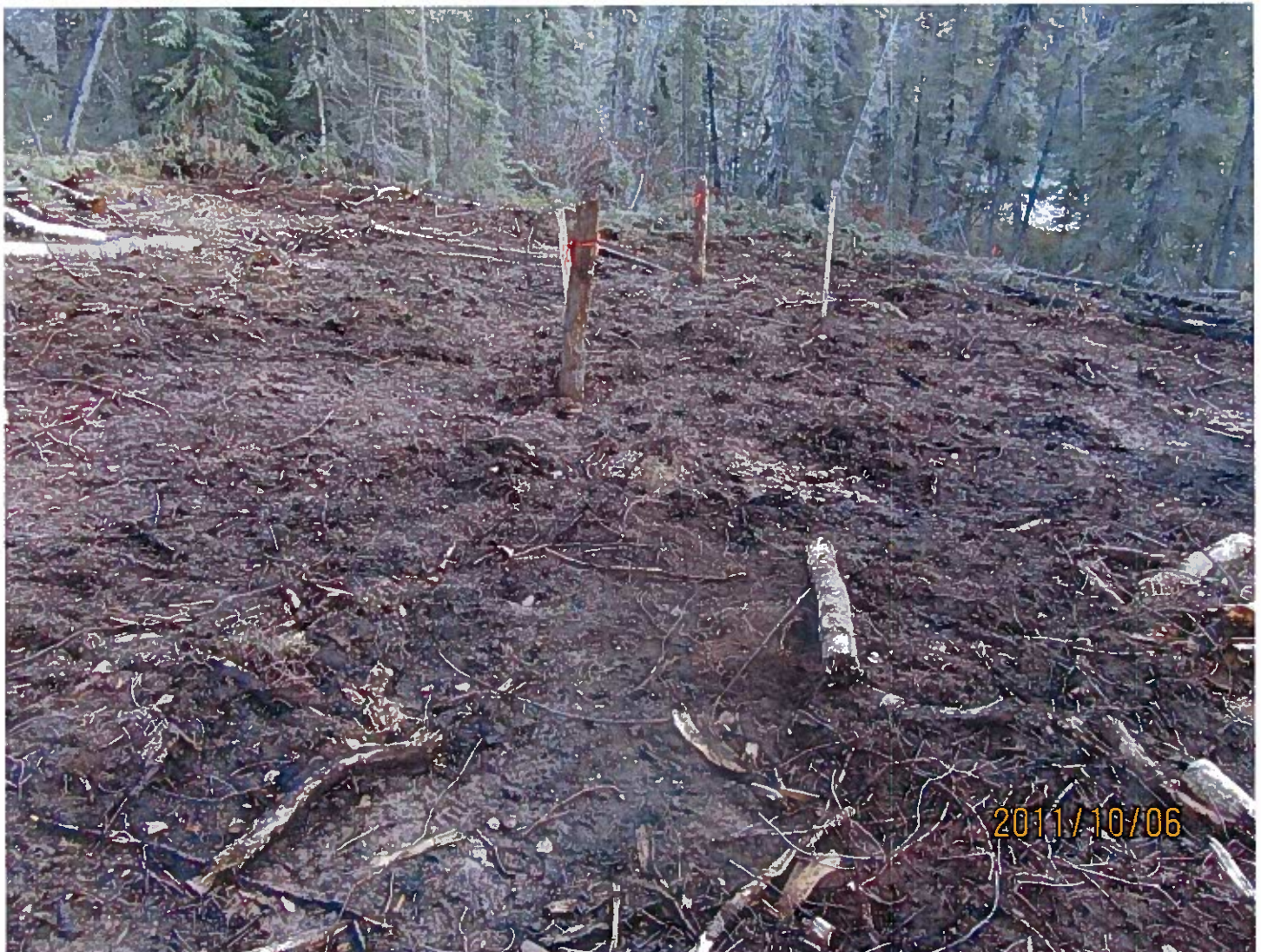
Photo #8 - Avalon Rare Metals Inc. - Thor Lake Completed drill site and the stick with flagging at the back of the photo has casing present that must be cut flush with the ground surface.
