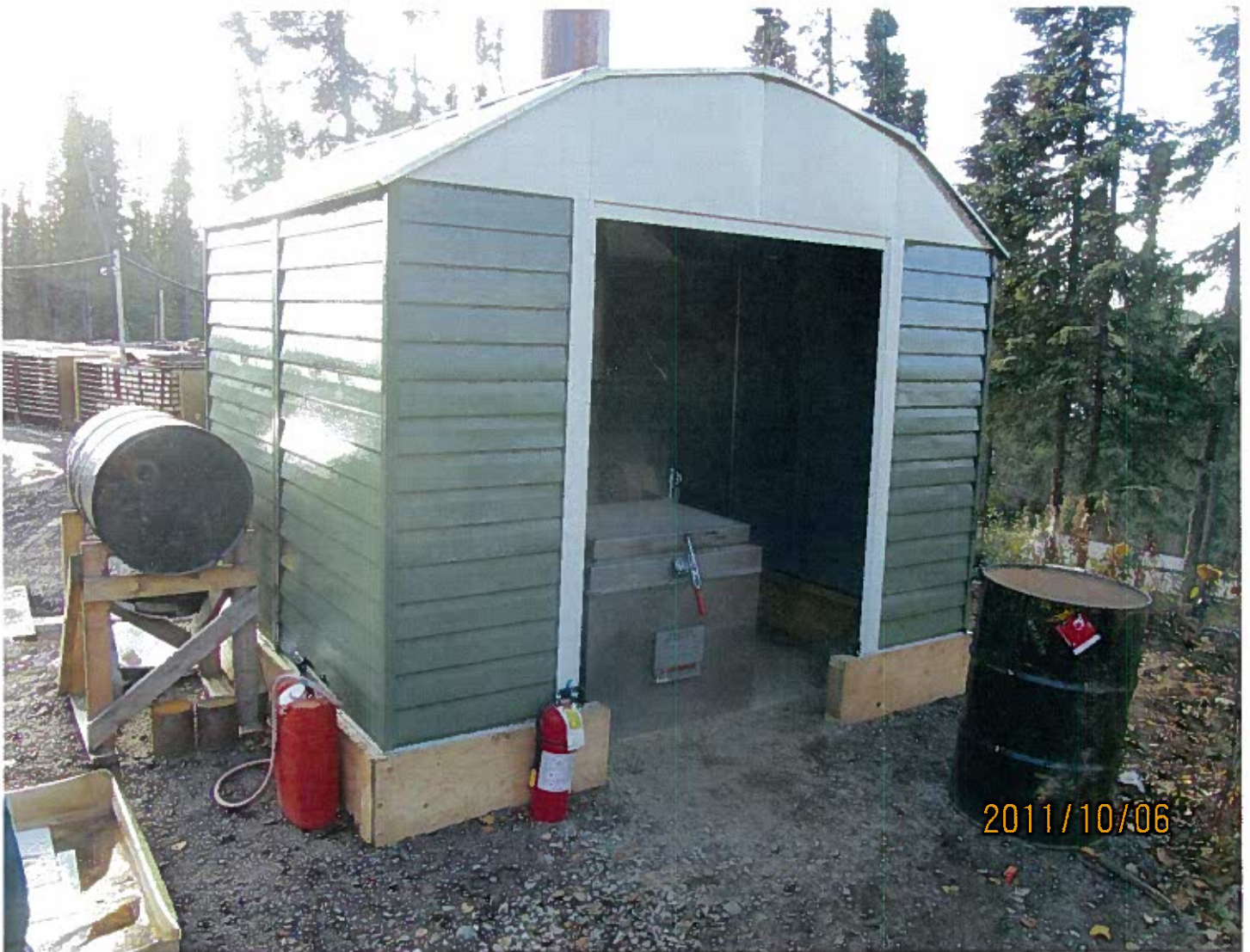
Photo #1 - Avalon Rare Metals Inc. - Thor Lake New incinerator at camp and it has a high temperature secondary burner.
