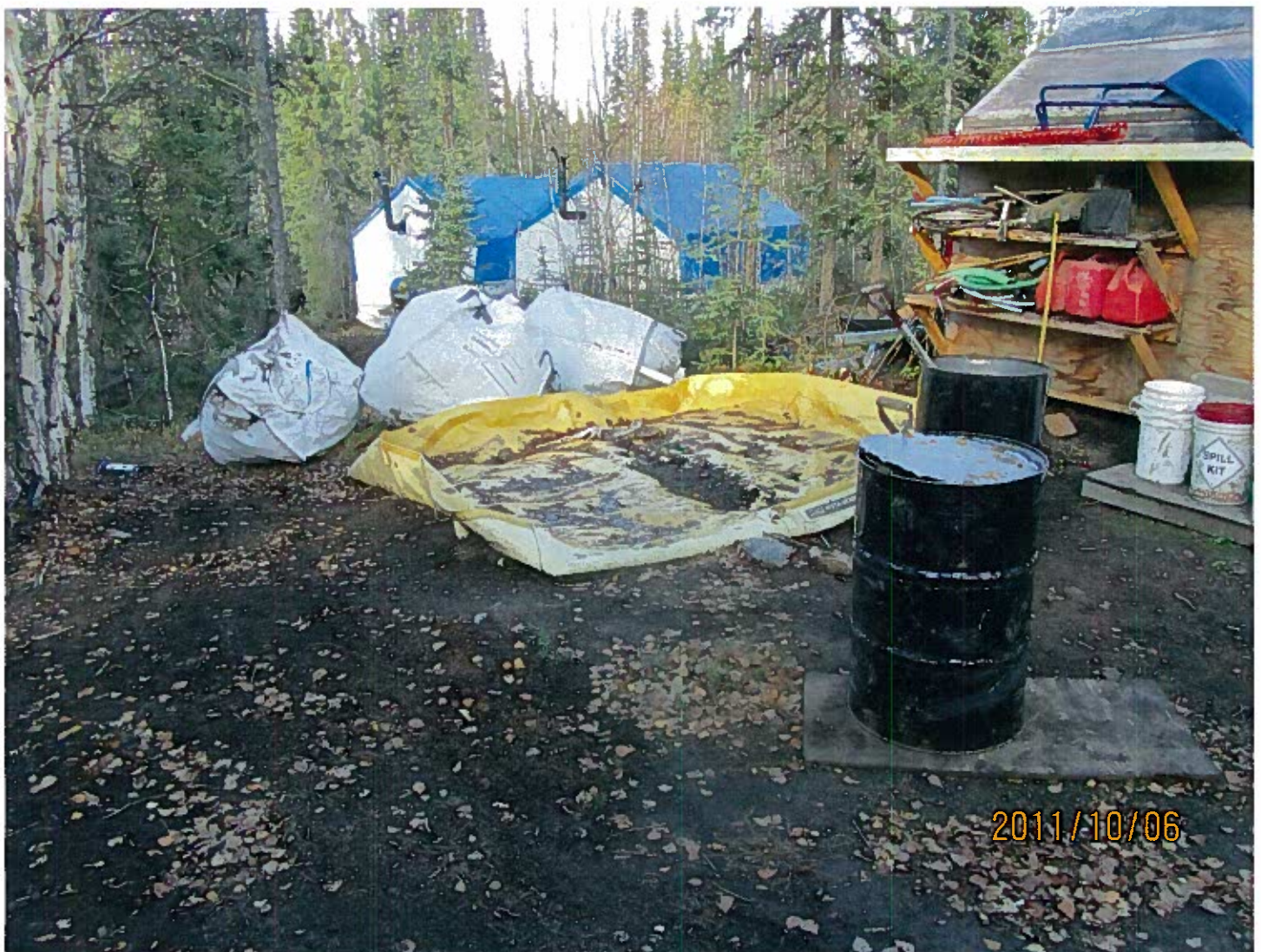
Photo #2 - Avalon Rare Metals Inc. - Thor Lake Hydrocarbon impacted soils were being land farmed in this instabern. They have since been containerized and shipped off site for disposal.
