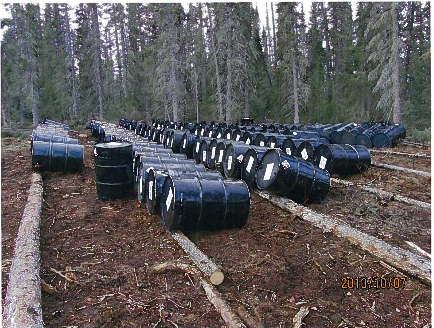
Photo #12 - Another well established fuel cache, and another good practice implemented by the Permittee. Drums have been slightly elevated by placing the top of the drums on logs.
