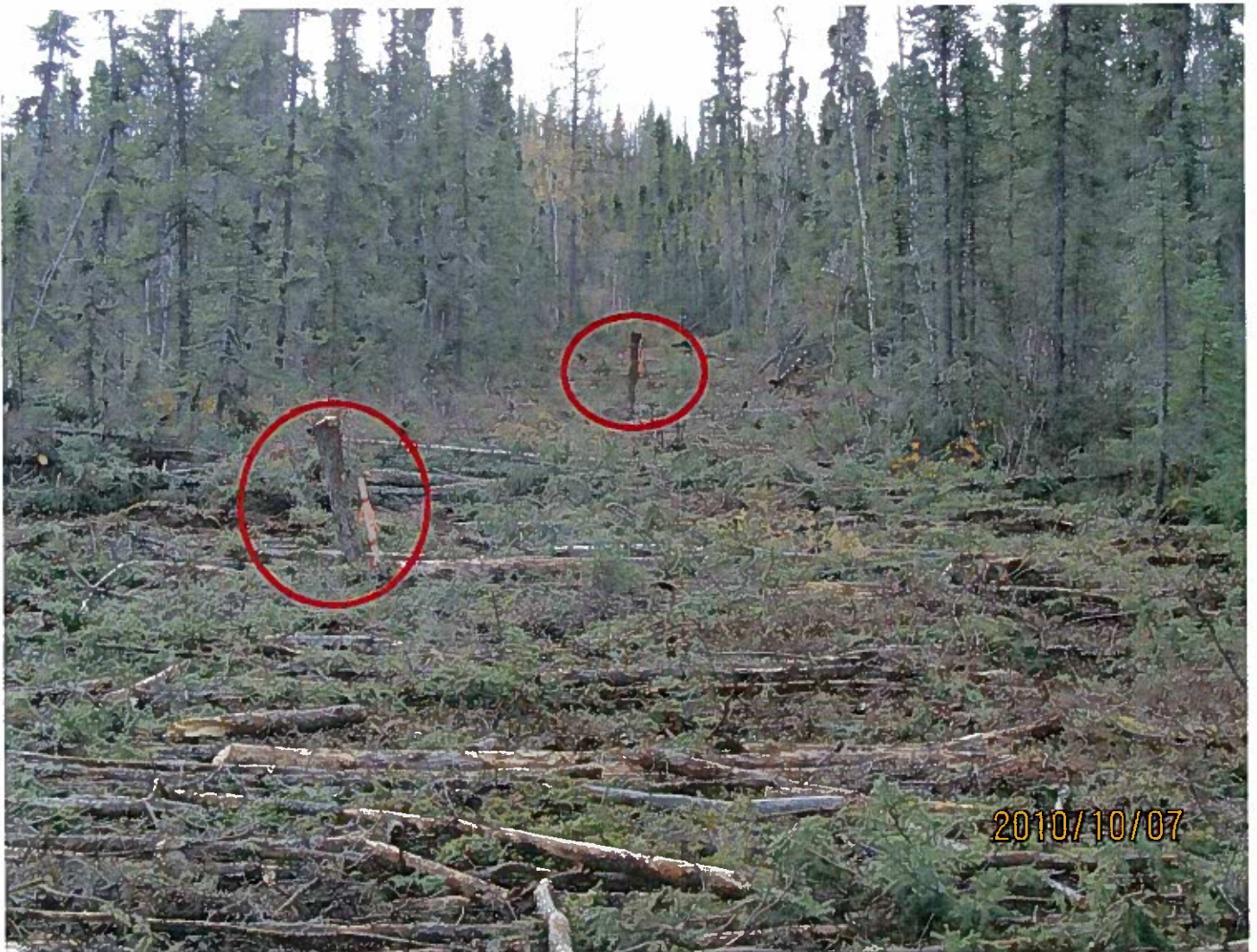
Photo #9 - Two completed drill sites (circled) and access trail are viewed in this photo. The Inspector was pleased with the reduction in clearing that occurred along this access trail, as trail width was a concern noted during the previous inspection.
