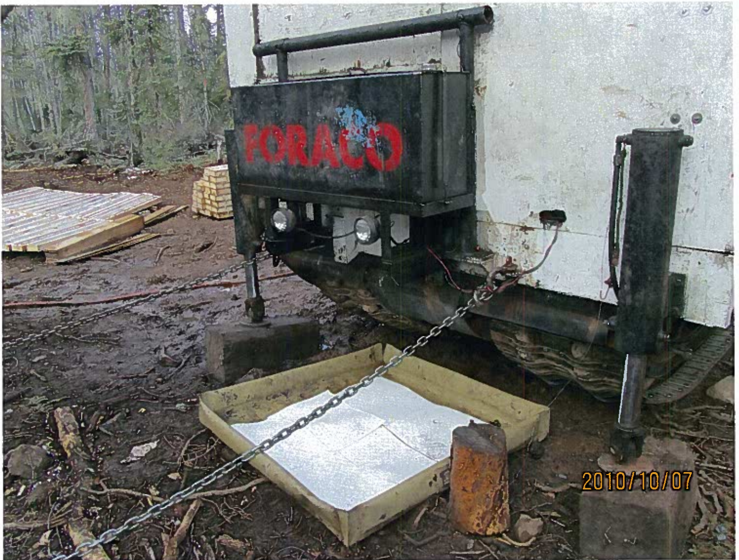
Photo #5 - Leaks/weepers from the fuel tank on the buggy drill has been a concern during previous inspections and the Inspector is pleased to report there were no concerns with it during this inspection and adequate secondary containment has been implemented.
