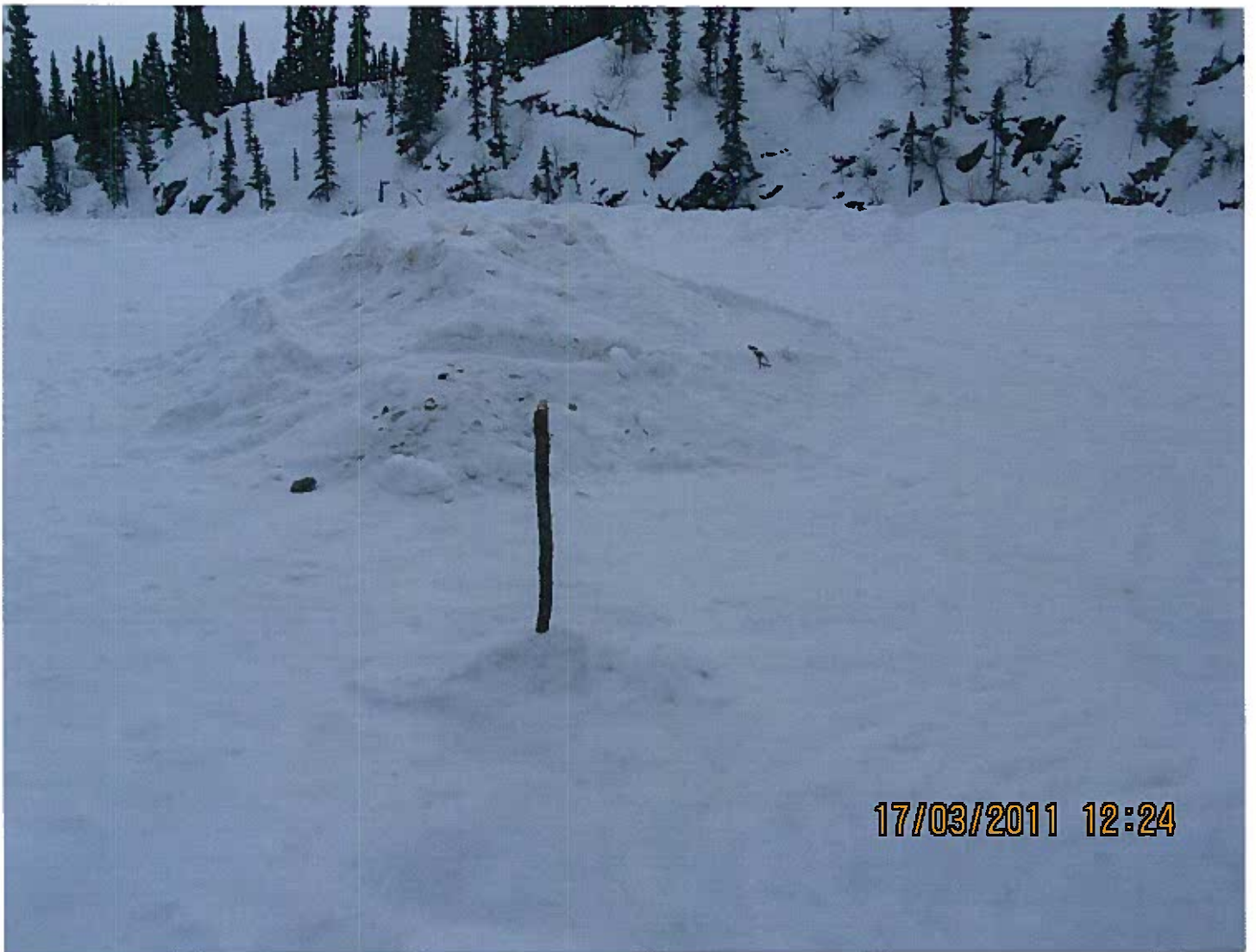
MV2007C0039 - Avalon Rare Metals Inc. - Mineral Exploration - Thor Lake, NT. Completed drill site on Long Lake. Pile of snow with some residual cuttings that will be transported to a land based disposal location.
