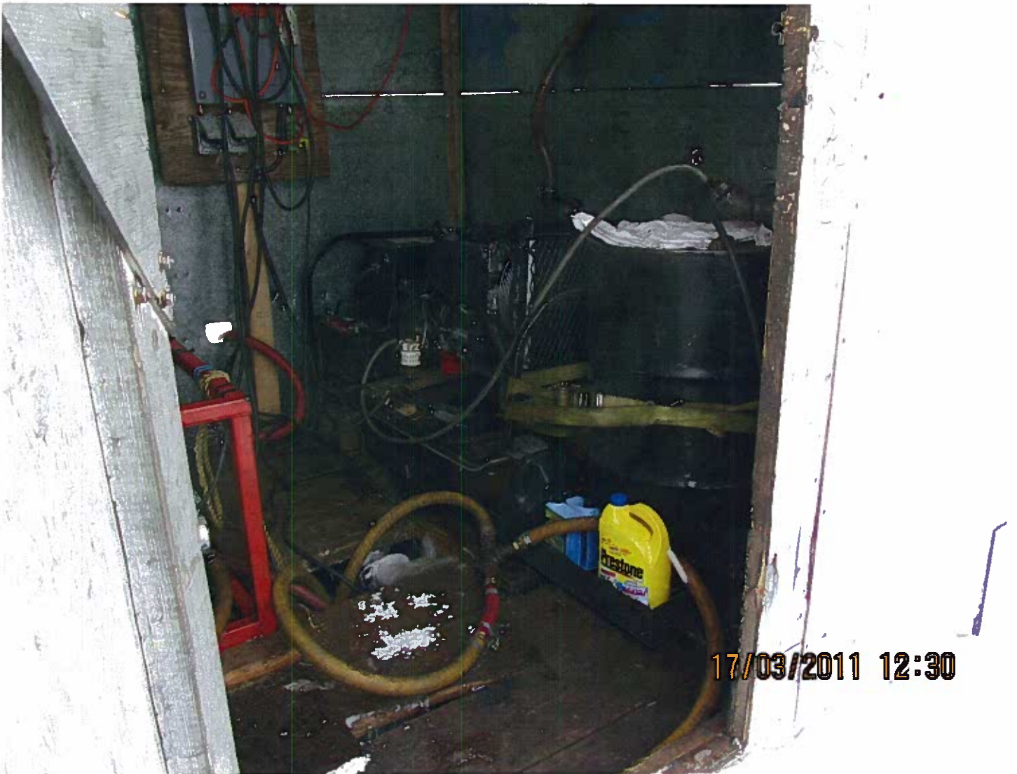
MV2007C0039 - Avalon Rare Metals Inc. - Mineral Exploration - Thor Lake, NT. Fuel at the pump shack is contained and absorbents were present under the pump.
